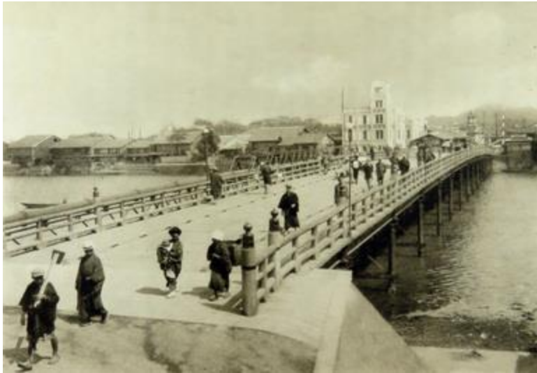
(写真左) The Long White Bridge at Matsue
