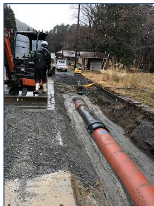
■水圧管は村道敷設 (L=1082.5m)
